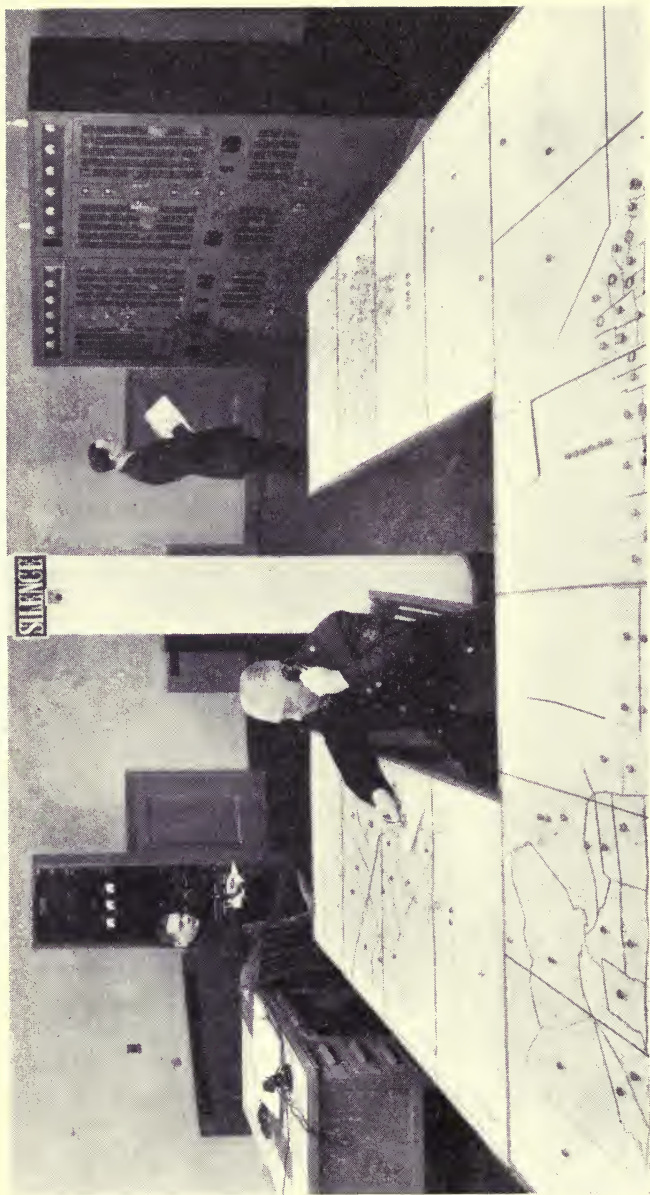
The nerve center of the New York City police radio patrol system. The dispatcher is surrounded by maps of the city's boroughs which indicate the location of all patrol cars on duty. Note, in background, transmitter at right, speech-input system at left.
